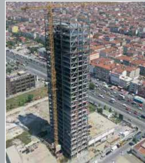
HILTON DOUBLE TREE (STEEL CONSTRUCTION) ISTANBUL
